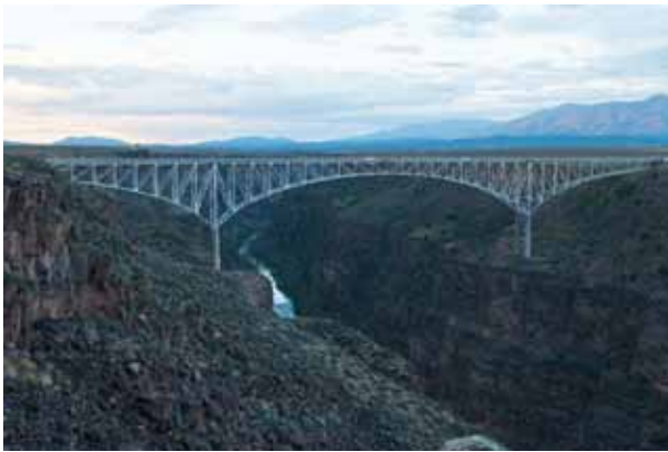
Rio Grande Gorge Bridge © Linda Martin
